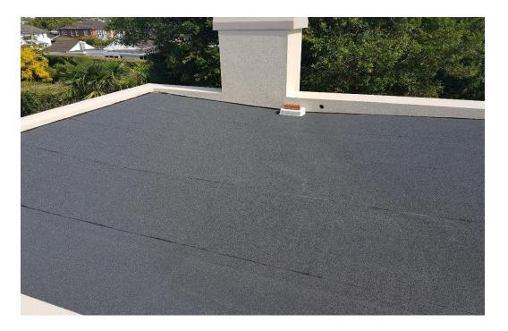
We gave the roof a high pressure wash and then proceeded to do all detail work and masking for the finish coat of Neptune Pacific Ltd OneCoat Grey, this was to be a finished dry film thickness of 1.5mm.
