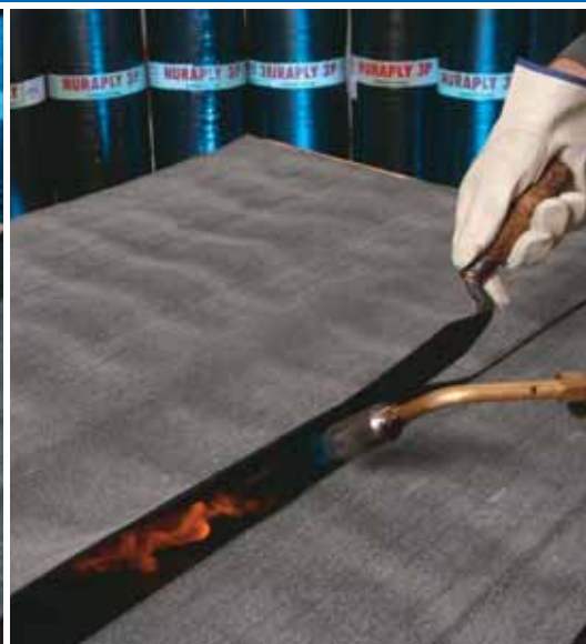
B/ Welding lap joints
