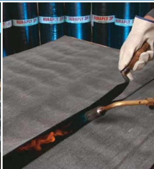
B (Welding lap joints)
