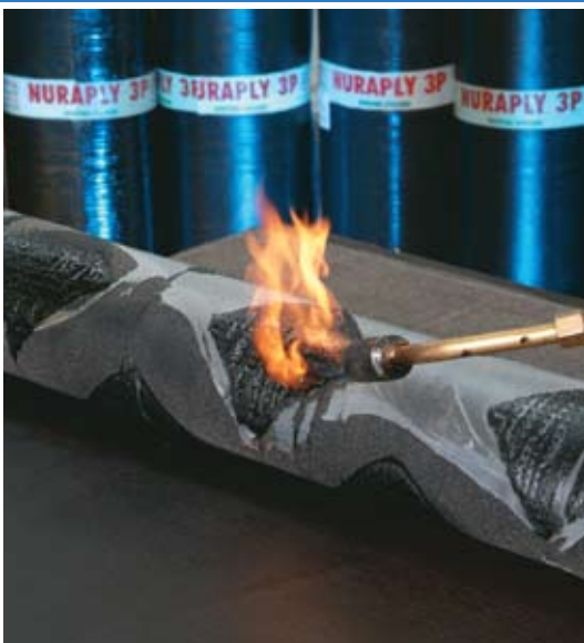
A (Melting bitumen adhesive pad)
