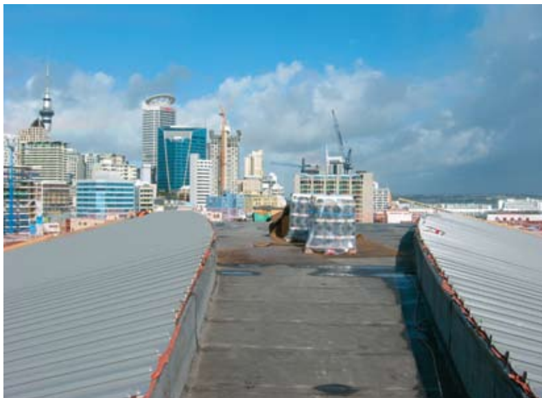
Vector Arena under construction, Auckland
