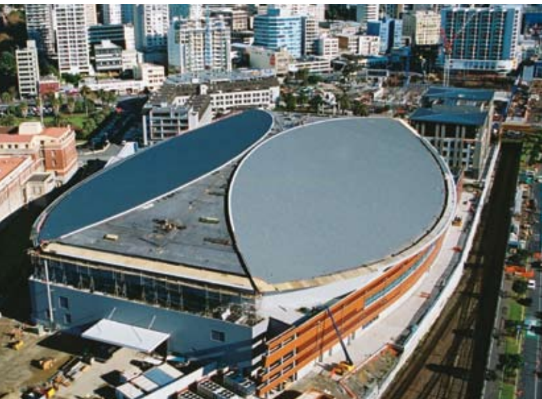
Vector Arena under construction, Auckland
