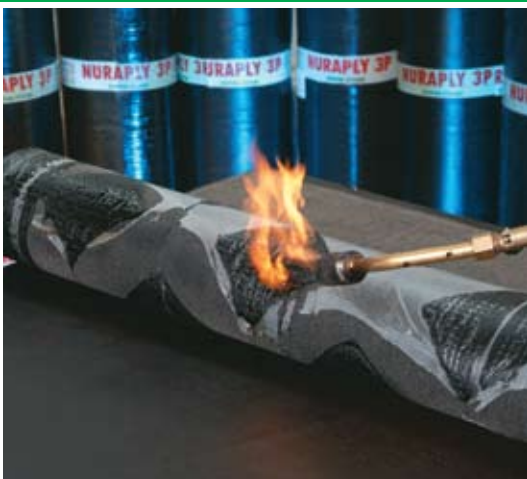
Melting bitumen adhesive pad
