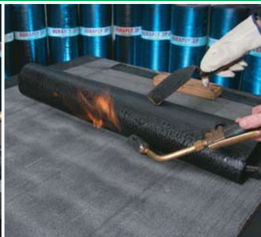
3PG heat welded to basesheet
