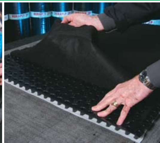
Drainage mat laid on membrane
