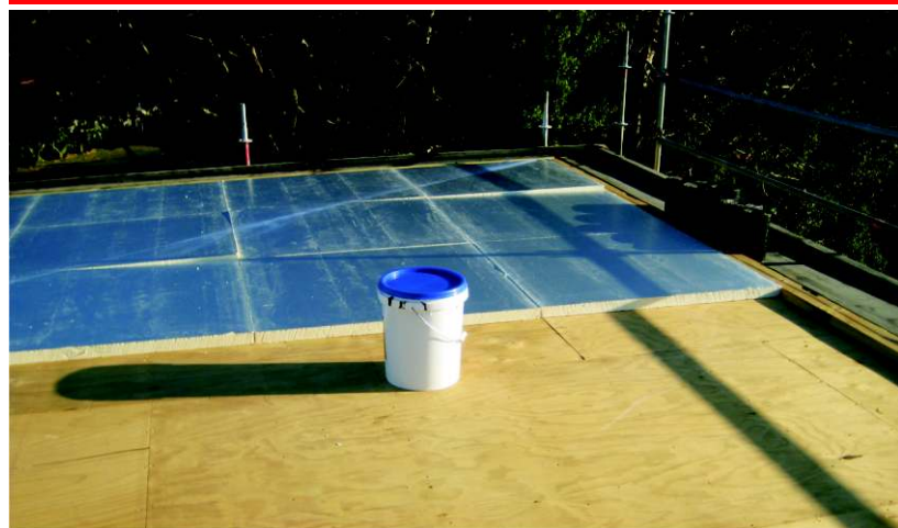
Insulation set out on plywood
