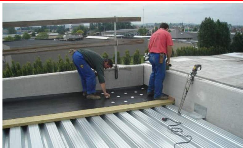
Insulation fixing on metal roofing
