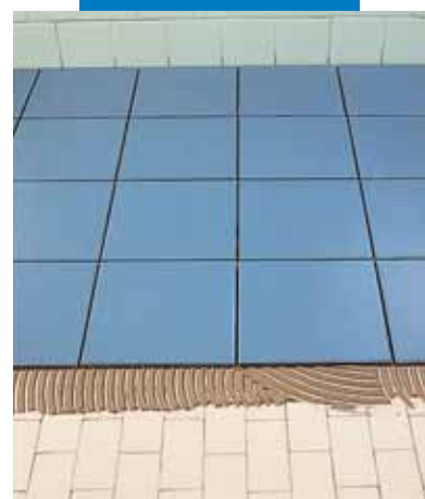
Tile on tile with Keraflex Grey
