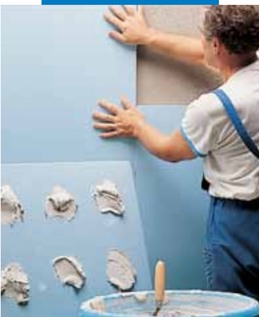
Laying polystyrene foam slabs with Keraflex white
