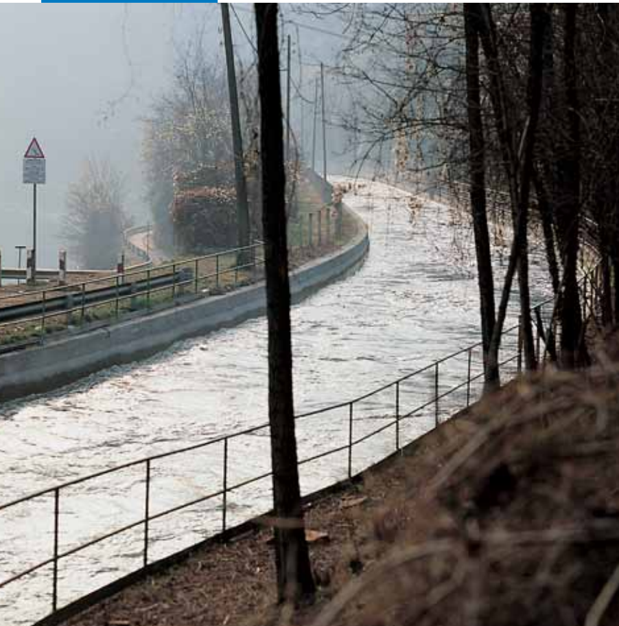
Bertini hydroelectric canal - Como - Italy. Surfaces treated with Idrosilex Pronto
