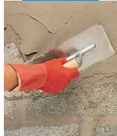
Application of Idrosilex Pronto by trowel
